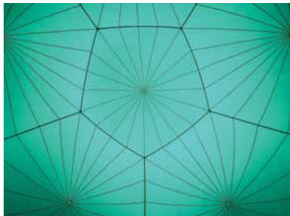
Above: Exxopolis seam detail design Centre: Exxopolis Red Dodecadome Below: Exxopolis Dodecadome seam pattern (interior) Photo: Lamar Francois
